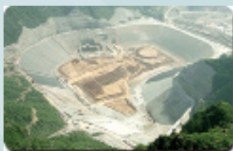
Baoquan Pumped Storage Power Project Upper Reservoir: Rockfill dam with asphalt concrete, H=94.8m Lower Reservoir: Masonry Dam, H=95m Installed Capacity: 1200MW
