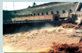
Sanmenxia Project Concrete Gravity Dam H=106m Installed Capacity: 400MW
