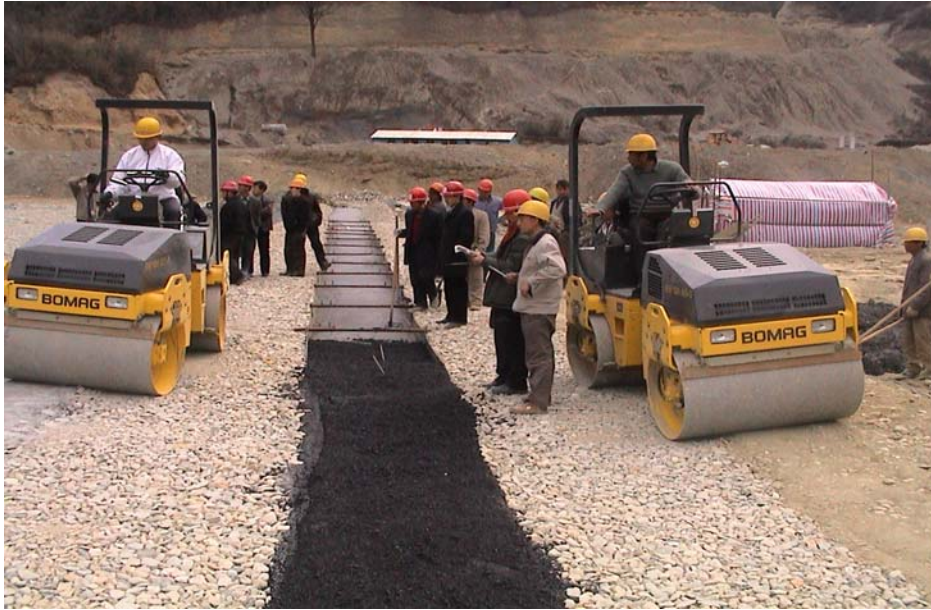
Fig.5 Site construction test of asphalt concrete (Upper Reservoir)
