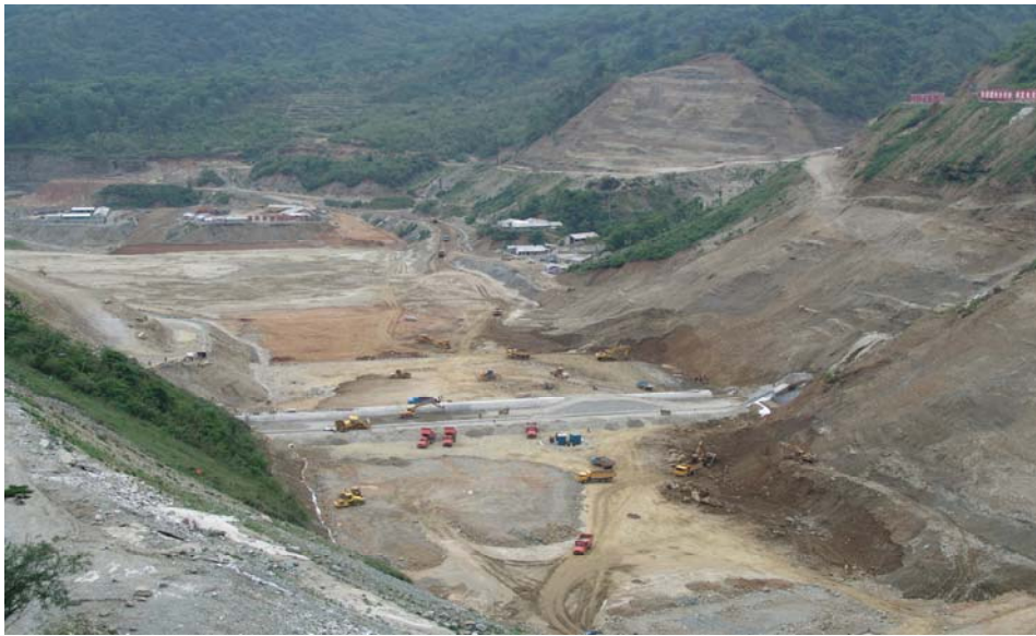
Fig.6 Rockfill construction of dam body (Lower Reservoir)
