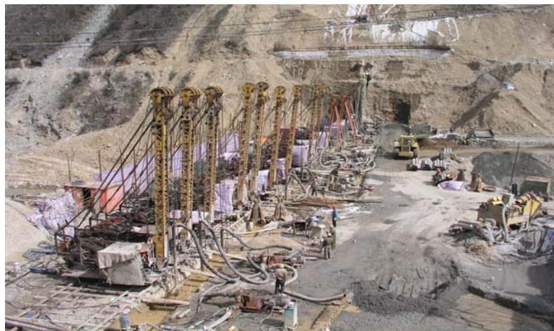
Fig.4 Construction of cutoff wall on river bed (Lower Reservoir)
