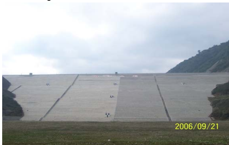
Fig.3 Downstream view of Yele dam of lower reservoir
