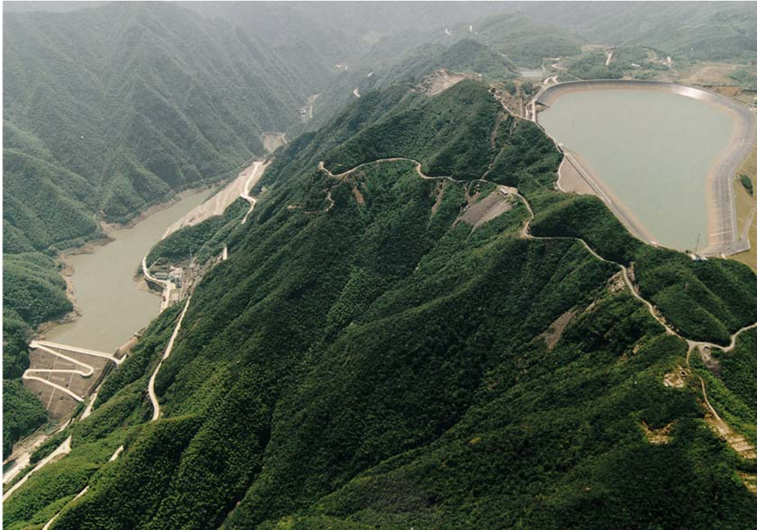
Fig. 1 Bird view of Tianhuangping Power Station
