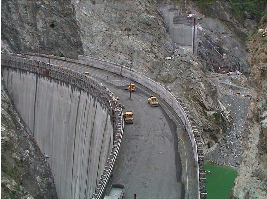
Fig.2 Construction of Shapai RCC Arch Dam
