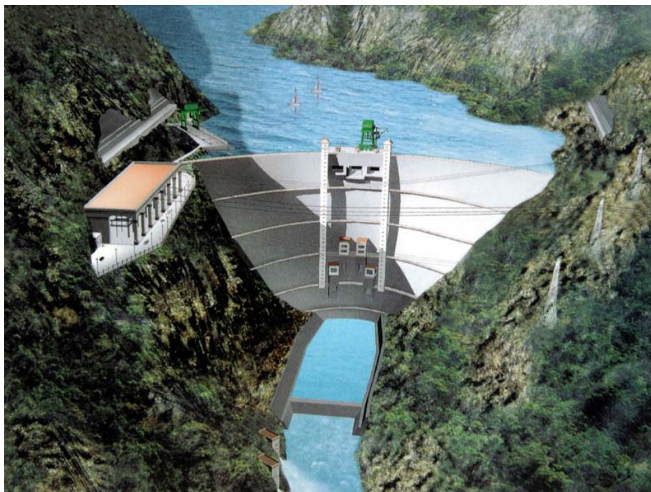
Bird's view of Laxiwa Hydropower Project
