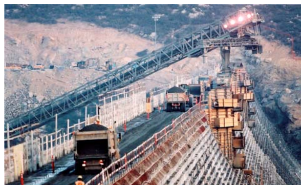
Truck on Dam (RCC Placement near Top)
