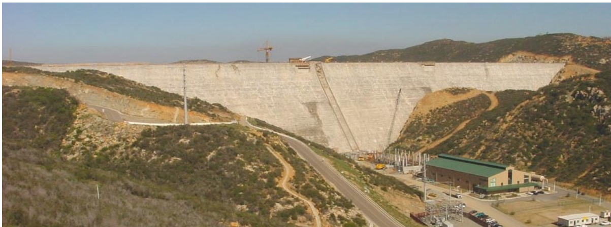
Downstream of Olivenhain Dam
