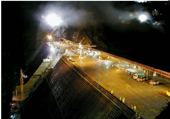
Construction at night (June 2003)
