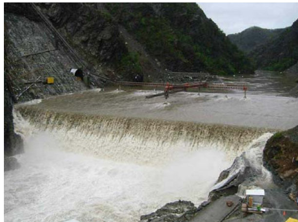
The second overtopping happened in October 2002
