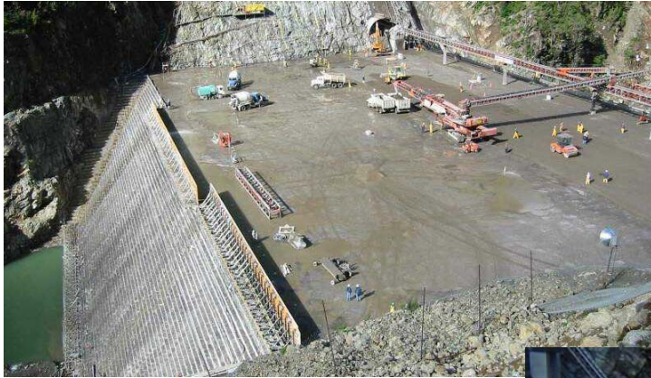
Re-construction in November 2002
