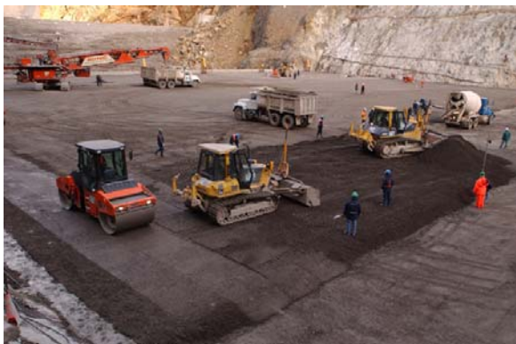
Bedding mix and Vibrating Rolling
