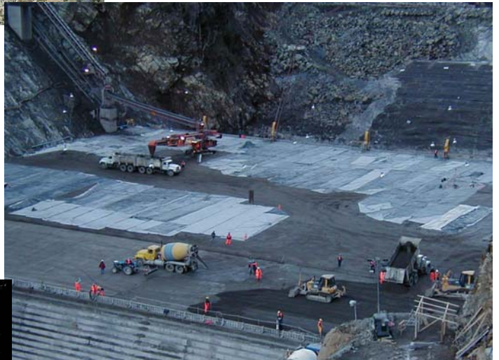
Protection of RCC exposed surface with thermal blankets
