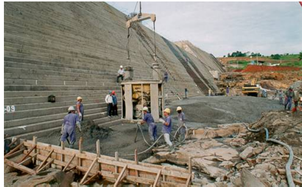
Downstream Rock Damages and Foundation Repairs
