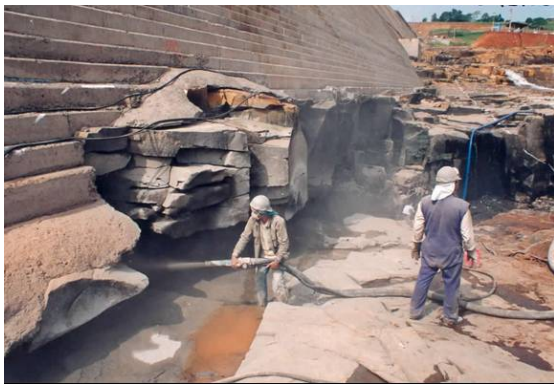
Downstream Rock Damages and Foundation Repairs
