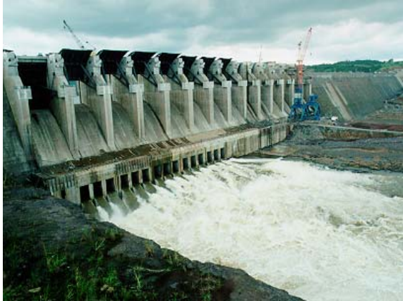
Sluiceways: downstream view
