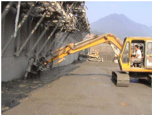
Vibrating of GEV RCC
