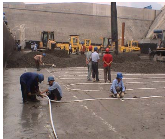
Laying PVC cooling pipes
