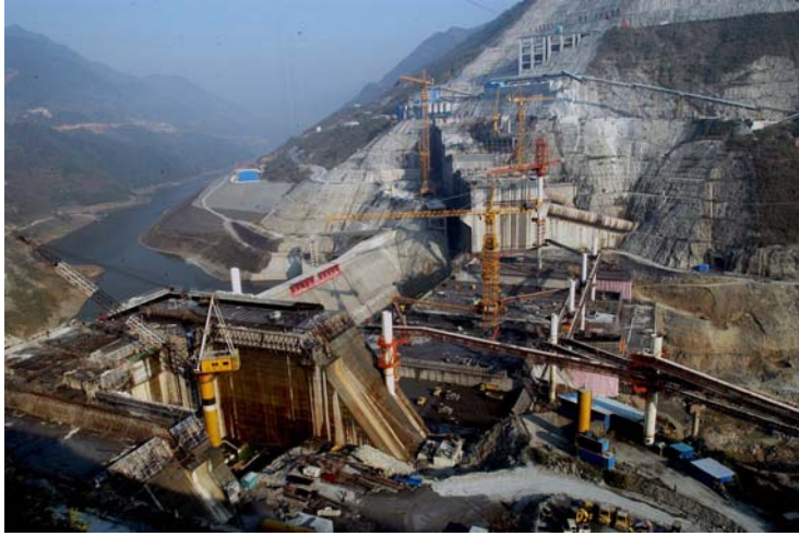
Construction Site of Longtan RCC Dam
