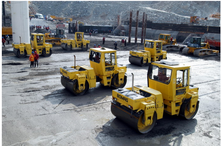
Constructed by vibrating rollers
