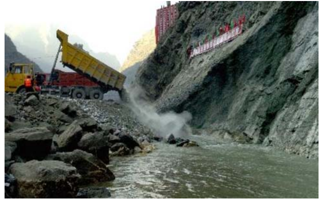
Fig. 5 River closure at Jinping I in Dec. 2006
