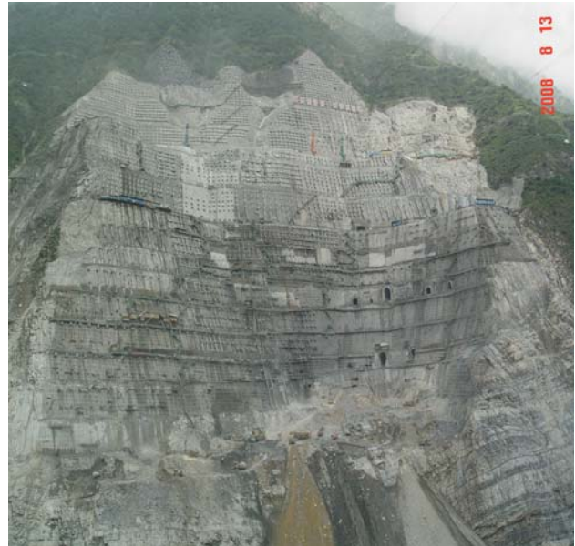
Fig. 17 Excavation of the left dam abutment of Jinping I
